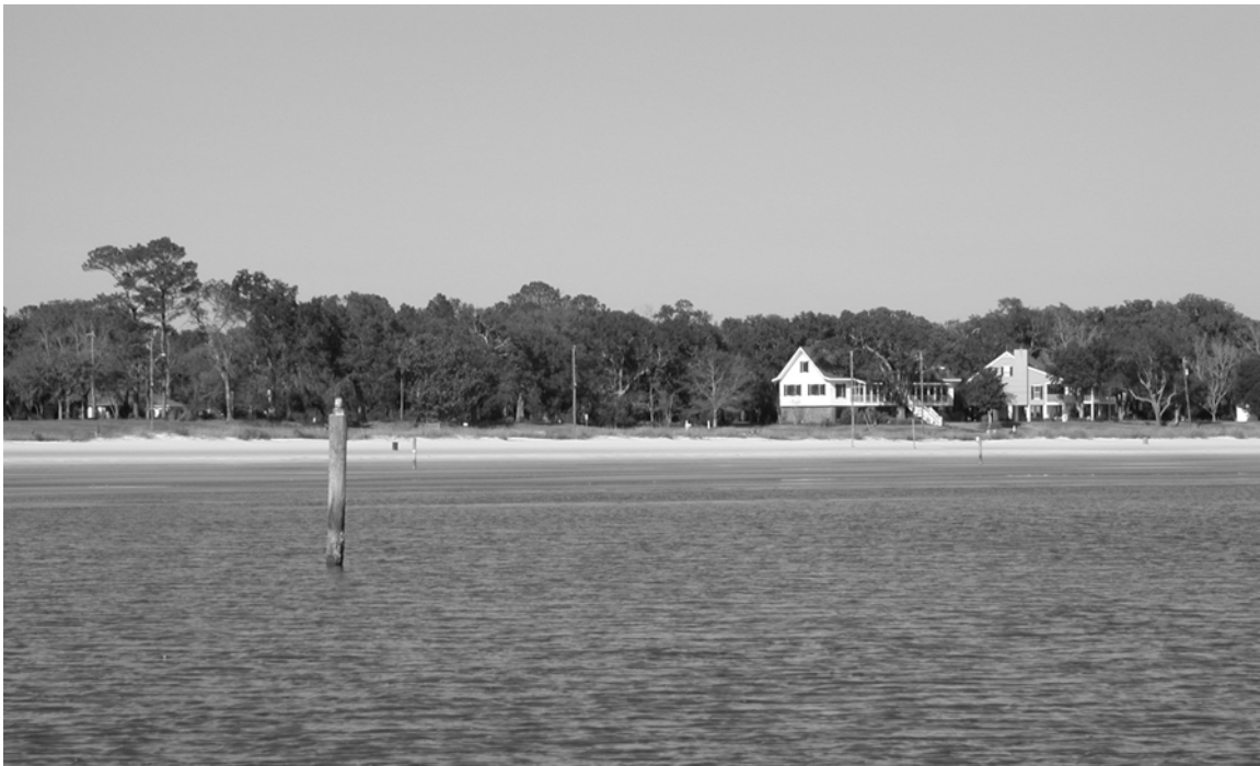
Picture 1. View towards shore from vessel anchored over borrow pit; piling is several meters shoreward of the actual borrow pit.
