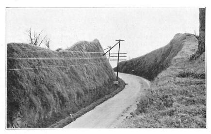
Figure 3.—Old Jackson Road cut into the Loess at the line of the Confederate trenches in the Vicksburg National Military Park. Although the verticality of the walls of the cut has been modified by recent improvement, nevertheless, the depth of the cut and the steepness of the walls are shown in this photograph of December 24, 1934.
