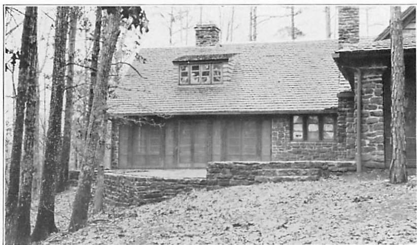
Figure 3.—North wing of Lodge, showing detail of native ferruginous sandstone construction.
