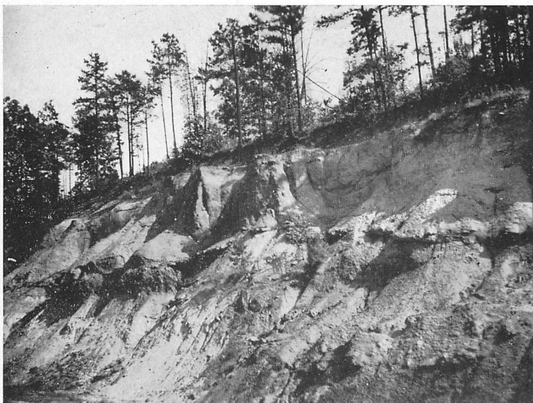
Figure 8.—Ackerman-Holly Springs faulted contact in the east wall of the Gulf, Mobile, & Ohio Railroad cut north of Williams Station.
