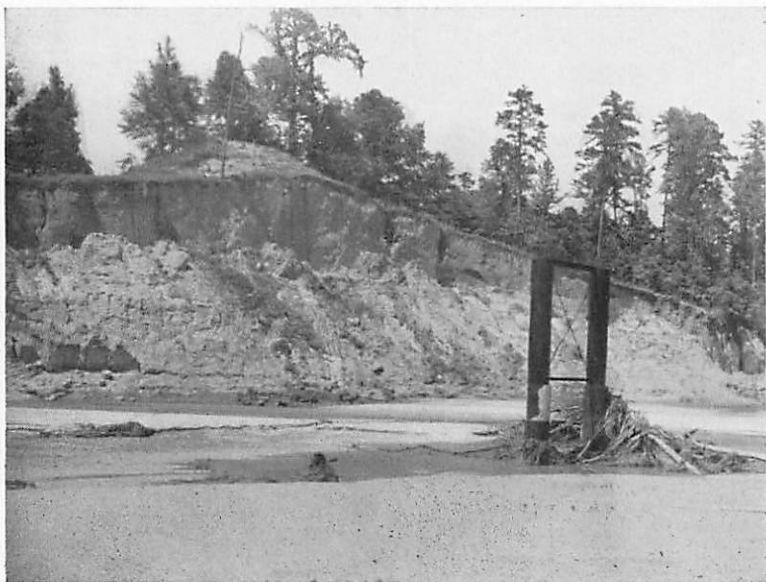
Figure 5. —Channel of Abiacha Creek (NE \frac{1}{4} , Sec. 13, T. 17 N., R. 1 E.) showing sand bars and pier of old bridge. Shipp's Creek shale crops out at foot of cliff just above water-level.
