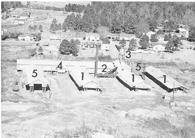
Figure 16.—Magnet Cove Barium Corporation's plant at Kosciusko: (1) dry shed; (2) rotary kiln; (3) grinding, screening and sacking; (4) storage; (5) rail or truck shipping facilities. Photo provided by Industrial Development Corporation.
