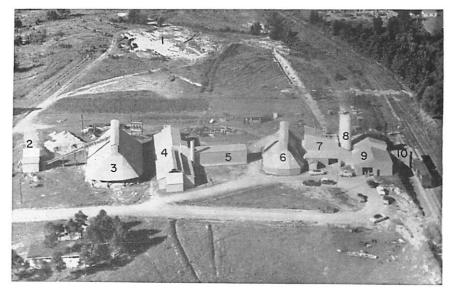
Figure 26.—Plant of Howell-Southern Products, Inc., Ripley, Tippah County, which produces fired clay aggregate for absorbent and deodorizing purposes: (1) clay pit—basal Porters Creek, (2) shredding shed, (3) dry shed, (4) kiln building, (5) cooler, (6) product storage, (7) screening and crushing, (8) silos, (9) bagging, and (10) loading. Looking south. (M.G.S. Bull. 86, Fig. 22). Richard Allin photo, December, 1958.
