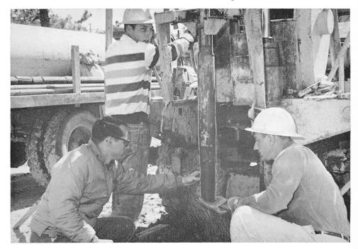
Figure 2.—Sampling of clay with the Survey's drilling rig using plunger-extruding core barrel. Note core lying on drill pipe on water truck. Photo by C. H. McMillan. March 5, 1964.
