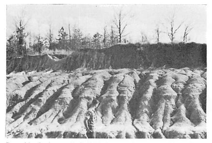
Figure 14.—Roadcut on U. S. Highway 80 near Clinton, Mississippi showing typical thin leached loess near to east margin. The loess rests on gray silty sand of the Catahoula (Miocene) formation (photo taken at sample station 22, figure 2).
