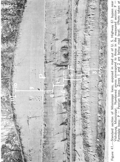
Figure 41.—Standard section of Mississippi loess, exposed in road cut of U. S. Highway 61 bypass near Vicksburg, Mississippi. Numbered zones correspond to those in the measured section: F = Farmdale loess; P = Peorian loess. Zones 1 and 2 are below road level. (Photo taken at footage 12,445, Figure 6).
