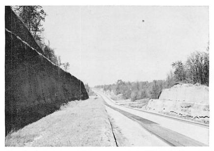
Figure 5.—Vertical, terraced highway cuts on U. S. Highway 61 bypass near Vicksburg, Mississippi.
