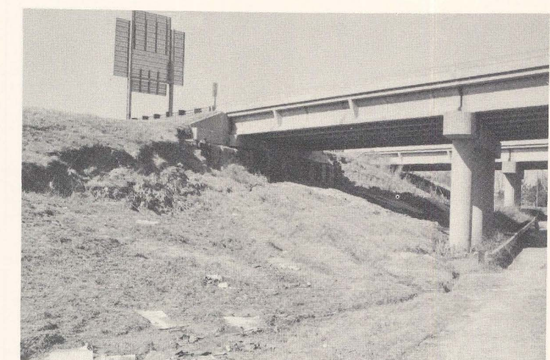
Figure 26. - Failure of bridge-end slope dictated remedial measures to save abutment. This structure built in Yazoo Formation outcrop belt.
