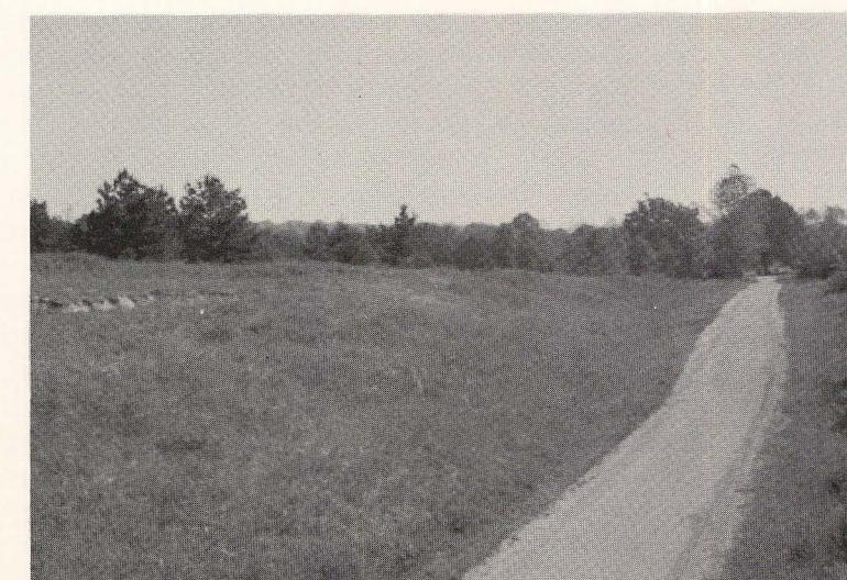
Figure 7. - Slump in clay of Yazoo Formation causing slight displacement of county road. Sec. 24, T.7 N., R.1 E., Madison County.
