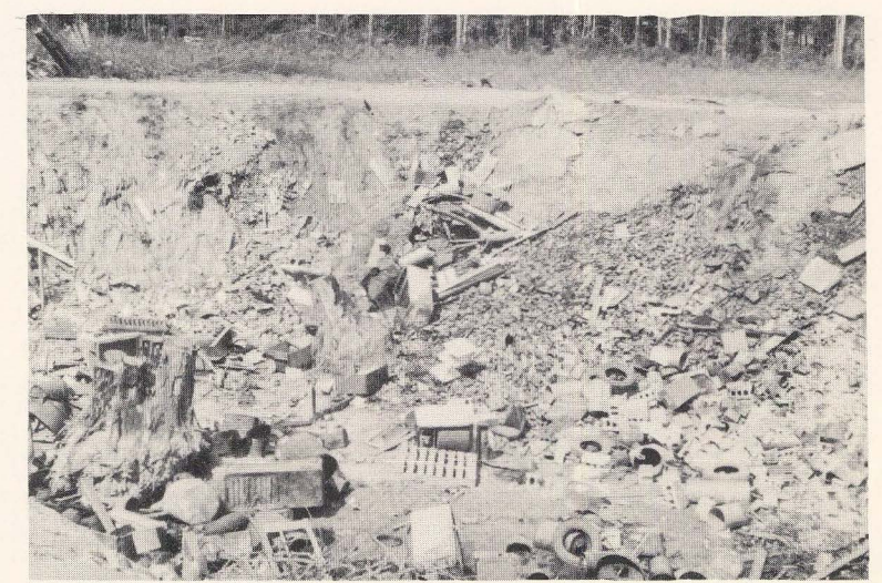
Figure 38. - Improperly managed trench landfill.
