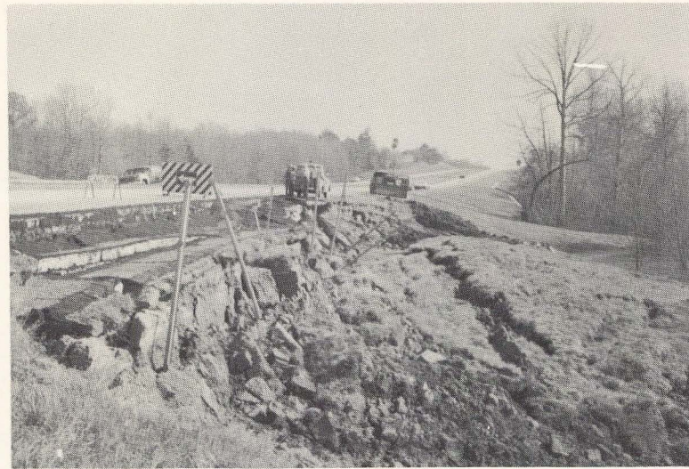
Figure 22. - Slump in Vicksburg Group outcrop causing damage to interstate highway.
