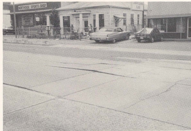
Figure 24. - Expansive Yazoo Formation clay causes numerous street failures in many of the towns in the study area.
