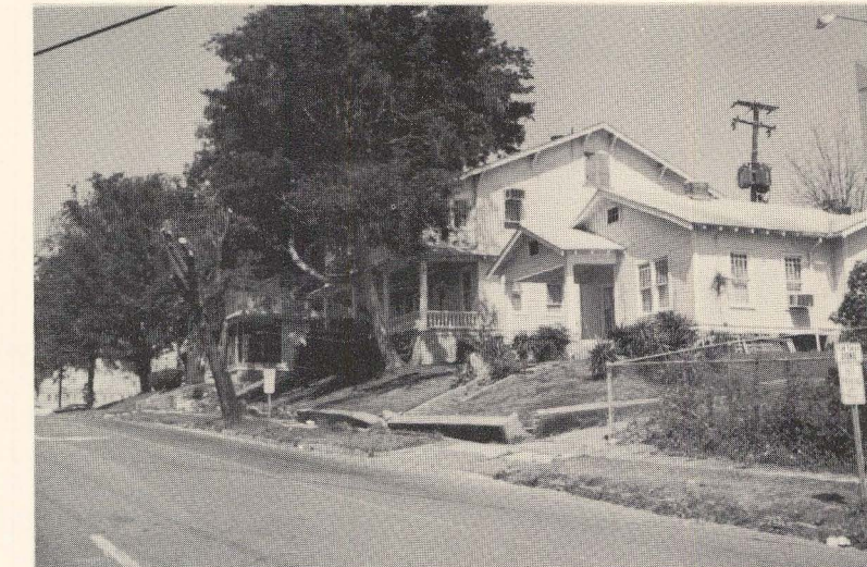
Figure 4. - Residences built on steep slope. Note leaning and broken wall and trees leaning because of soil creep.
